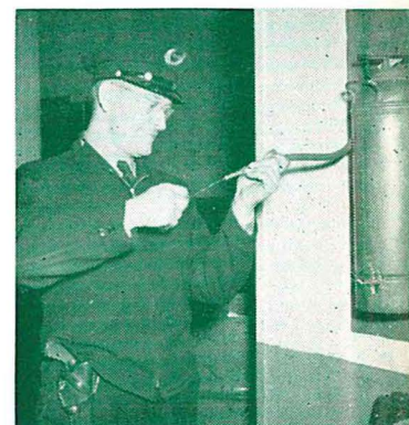
Thoughtless employees sometimes plug the fire extinguisher hose. Guard Charles Raderstorf checks opening on this extinguisher.
